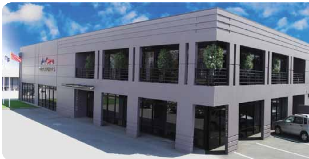
AuCom manufacturing plant in Christchurch, New Zealand.
